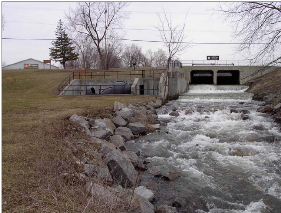
Photo 5.1- Sydenham Lake Dam Outflow, April 2002 (CRCA, 2005)
